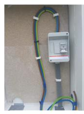
(533.3.5) A main overcurrent protective device may be located within a standard meter cabinet, in which case it shall comply with the following requirements:
