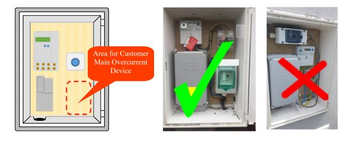
Again we are highlighting problems we are finding on domestic installations when interfacing with the ESB, below is the rule requirement when the Main Overcurrent device is located in the meter cabinet.
