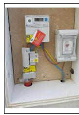
There is a ESB issue here as an isolator has not been provided, please report this to the ESB if you come across this type of connection. Also the Main Overcurrent device should have been located tighter in the right hand corner as we are finding in some areas a CT enclosure is being fitted and room gets very tight.
