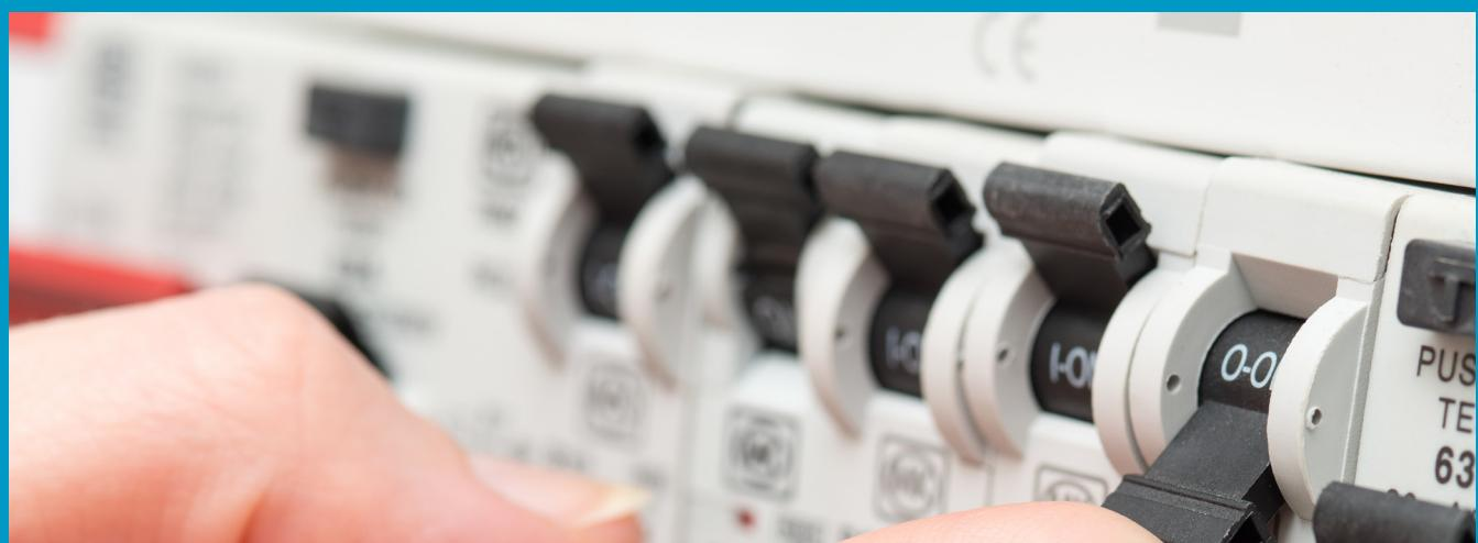
As we are dealing with AC and the RCD, response time can vary at different sides of the sine wave, we are obliged to carry out each test at both the top and the bottom of the sine wave. Therefore, we are required to test the device twice at each parameter and record the highest (Worst Case) reading. This is done by using the 0- and 180-degrees function on the test equipment. These requirements are outlined in Annex 61G of the current wiring rules.
